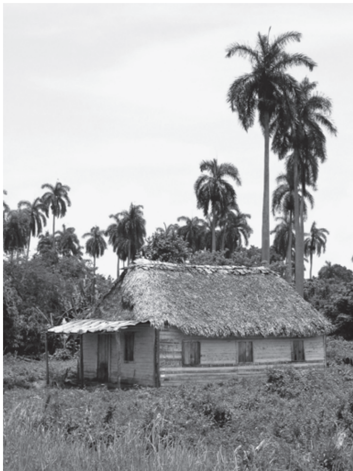
FIGURE 1.7. Typical rural dwelling made of palm thatching, palm wood (sides), and a zinc roof modification on front porch, Ciego de Avila Province, 2003.
